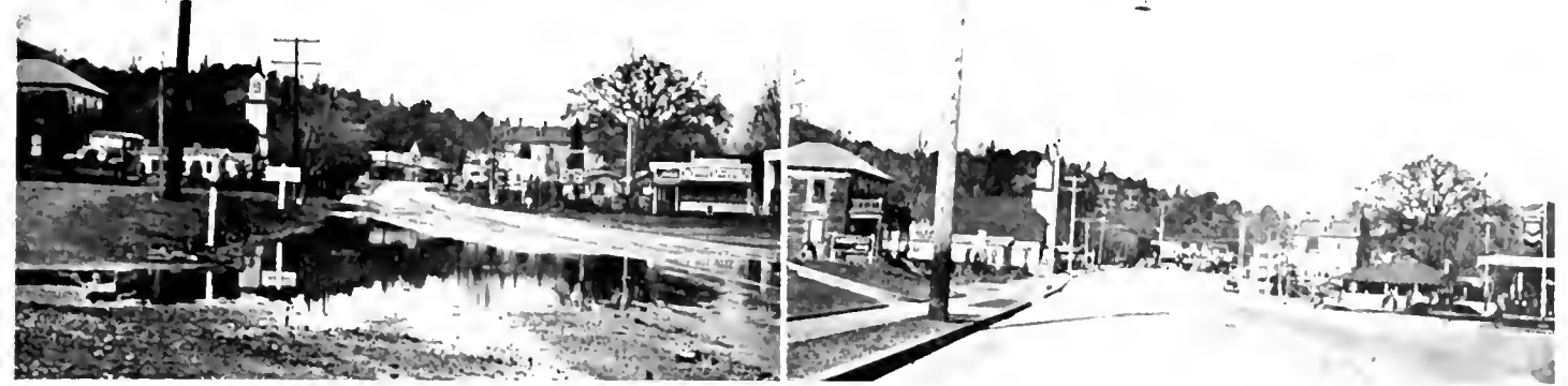
Before and after views on recently improved section of Redwood Highway in the city of Hopland
